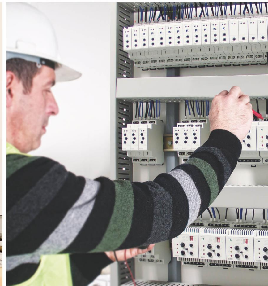
Realization support on site
